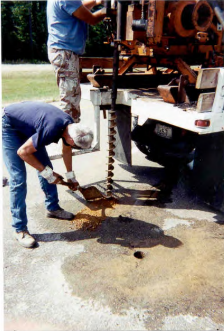
Figure 3.2 (b): Drill Rig Used for Sampling
