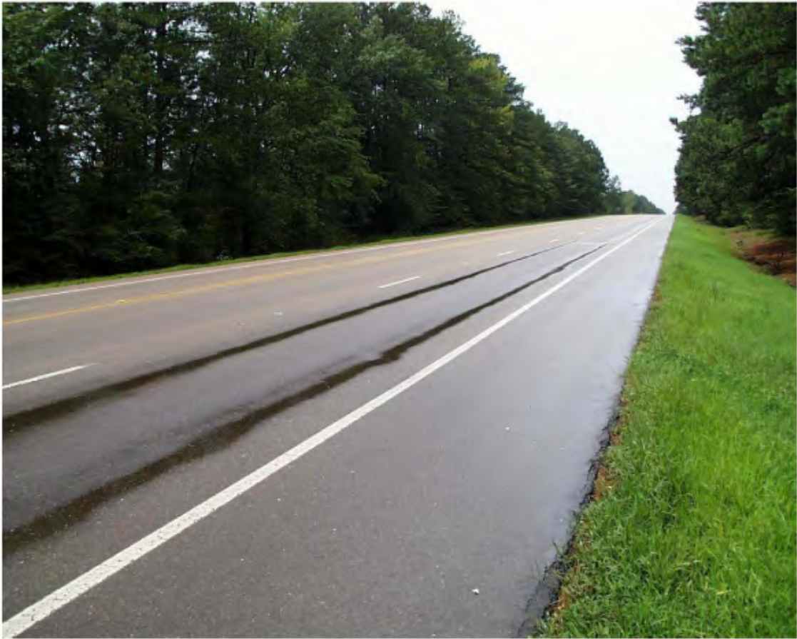
Figure 3.4: Rutting Along Highway 82
