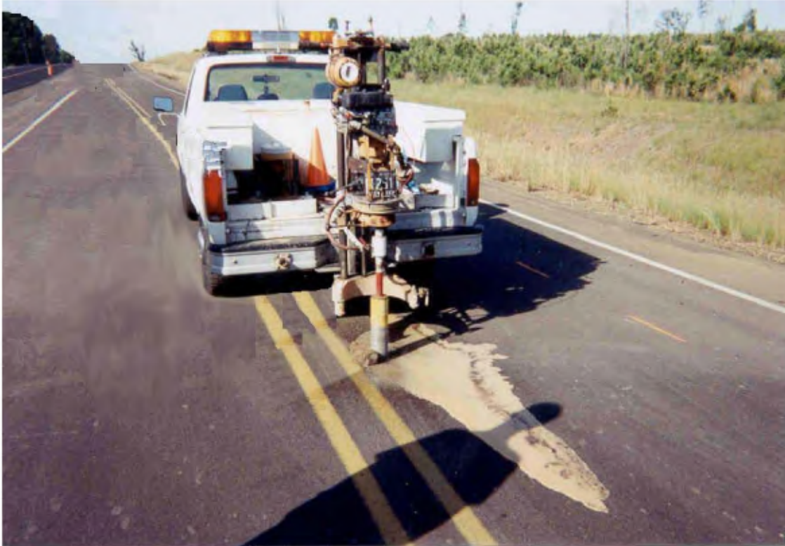
Figure 3.2 (a): Asphalt Coring Equipment
